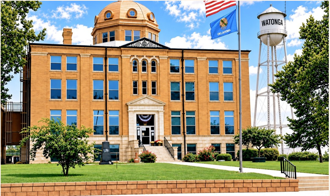
The Blaine County Courthouse — one of ten stops on the coming historic walking tour.
